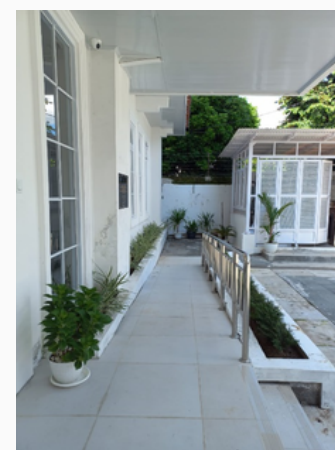
Ramp for users with wheelchairs
