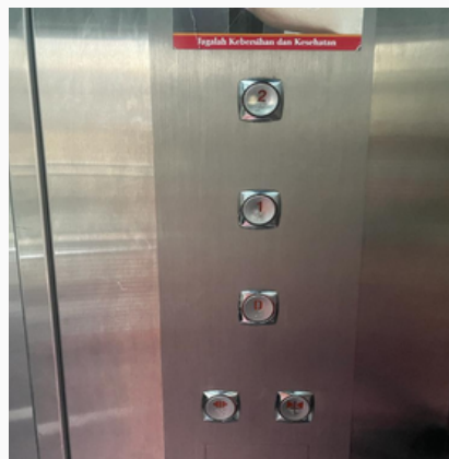
Elevators with buttons and signs in Braille
