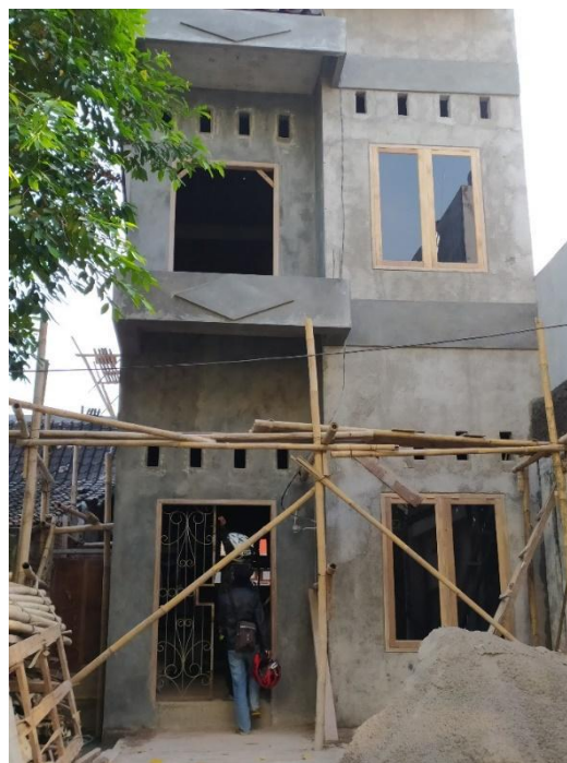
Figure 4. Roof heights and terrace distances are not yet compliant
