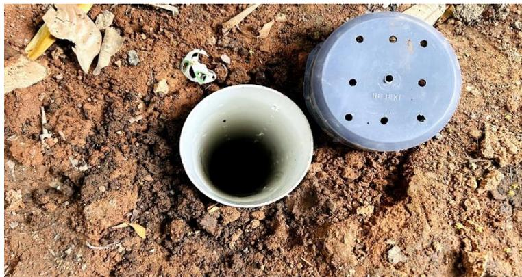
**Gambar 7.** Lubang Resapan Biopori (LRB) program KKN 172 Desa Cihanyir
