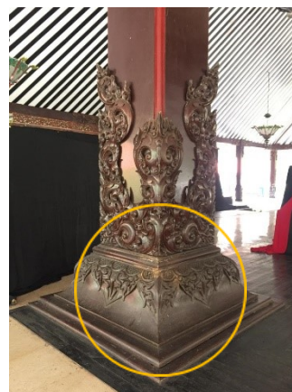
Gambar 7. Umpak Pendopo (Sumber: Survei, 2021)
