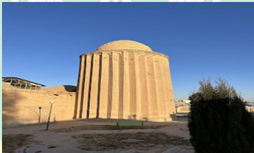
Gambar 19.4: Menara Khasaneh. Sumber: https://cyrus49.wordpress.com/2017/07/12/kashaneh-tower-by-aban-chinoy/ .
