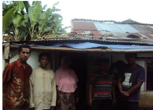
Home Condition of Mr. Aswidi (12 March 2016)
