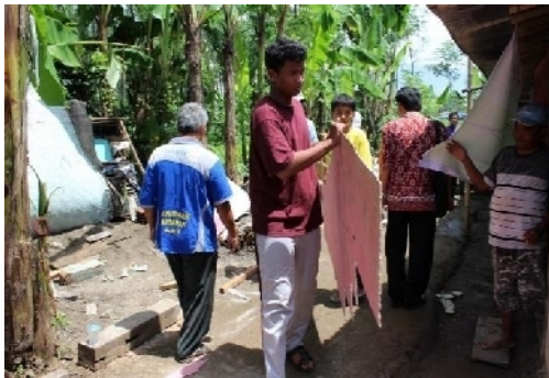
The renovation of the wall in the Benah Rumah Program (16 March 2016)
