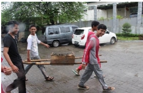
The Students Bring The Building Material to The Location of PLM (16 March 2016)
